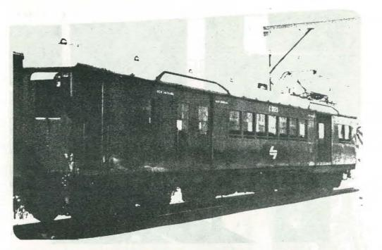
PHOTO 1. Lovely old Granny EMU, 60 years young, but still spry! C 3223 was serving as shop switcher here. Paint is Tuscan Red, with Yellow lettering and white 'L7' symbol. Roof is Silver, underframe black. Handrails are natural brass, except elbows, which are Tuscan. Interior is Green, the first 24" mid-green, light green above, including ceiling. Seats are deep green, with light brown floor.
