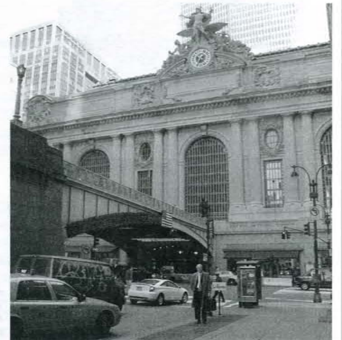
David Howarth standing near the Park Avenue viaduct, at the East 42 Street face of Grand Central Terminal.
