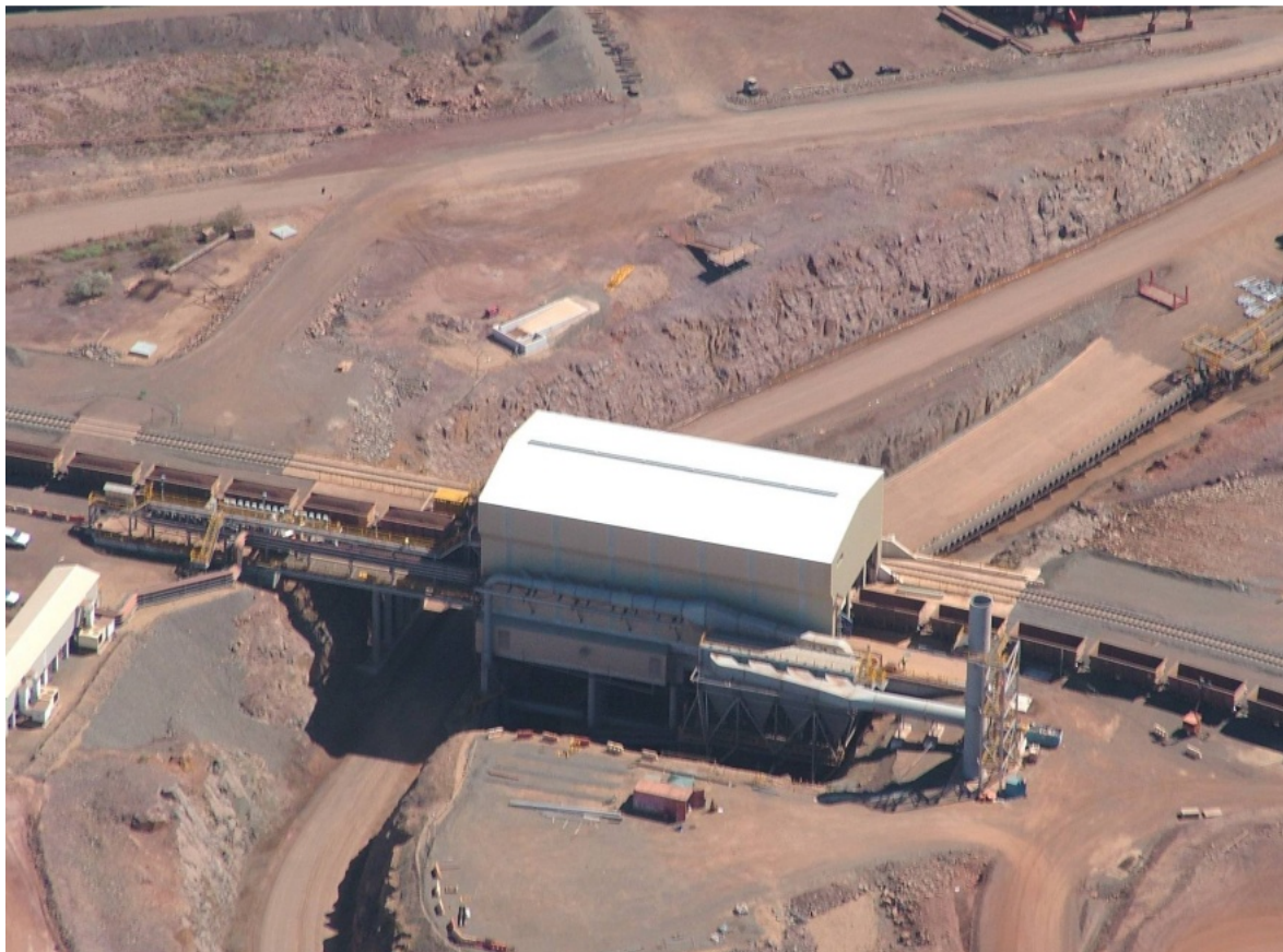
Photo 5 – Is the completed Car Dumper facility from the South with a string of wagons being unloaded moving from the left to the right.
