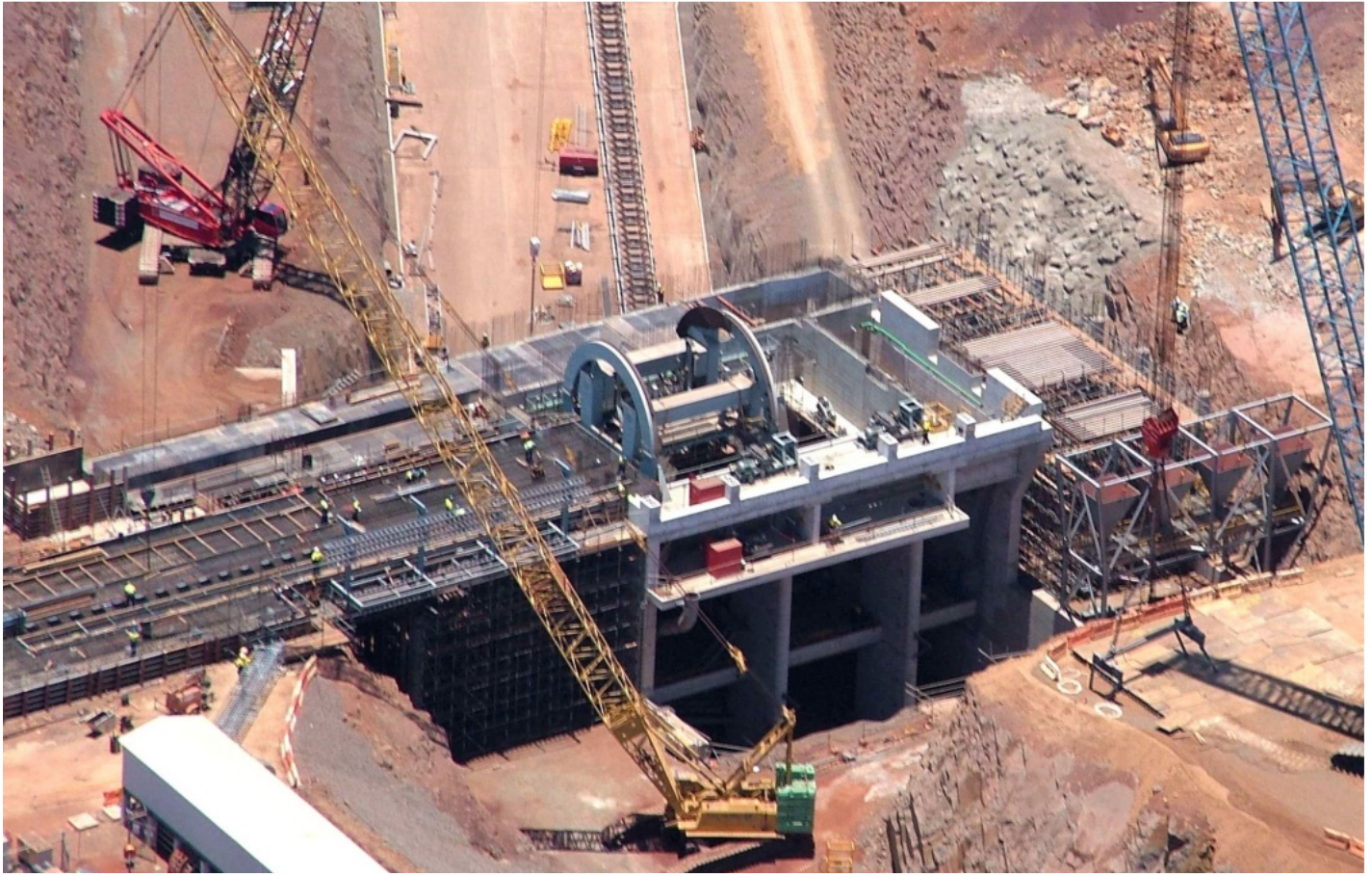
Photo 4 – A view of the Car Dumper from the South. One of the cells is in place with concrete structures prepared to the right for the second cell. Track bed is being prepared for entry into the cell from the left, and to the top left of this is space for track for empty wagon movements. This is shown more clearly in Photo 5 below.
