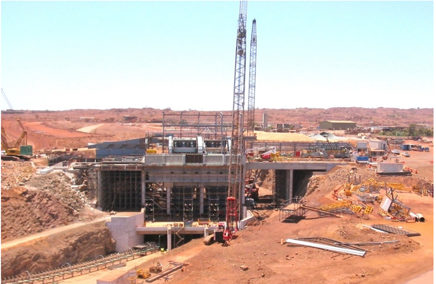
Photo 2 – Shows a view of the Car Dumper, from the North part way through construction. Note the two cells on the upper level which are the rotating sections of the dumper and the out-loading conveyor leaving the dumper from bottom left.
