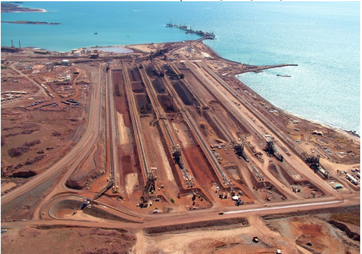
Photo 1 – Hamersley Iron –Parker Point Port Facility, Dampier (part way through recent construction) The car dumper is the white building in the top left hand corner just below the cluster of tanks on the coast. The balloon loop serving the car dumper can be seen sweeping off the page to the bottom left. The stockyards are the long strips running up and down the page holding the iron ore. The wharf can be seen in the centre top of the photo.
