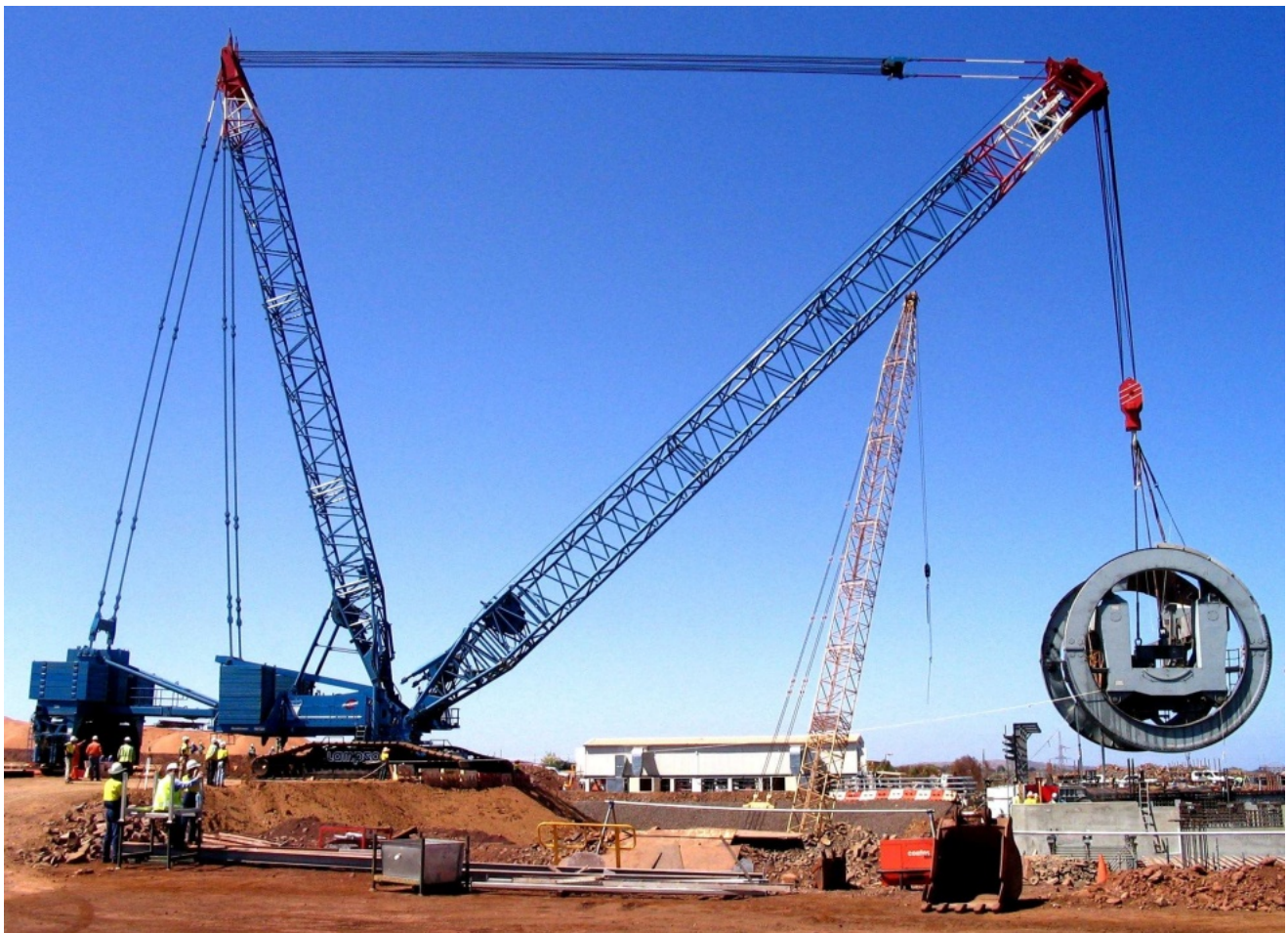
Photo 3 – Shows a Car Dumper Cell being lifted into place on prepared concrete foundations.
