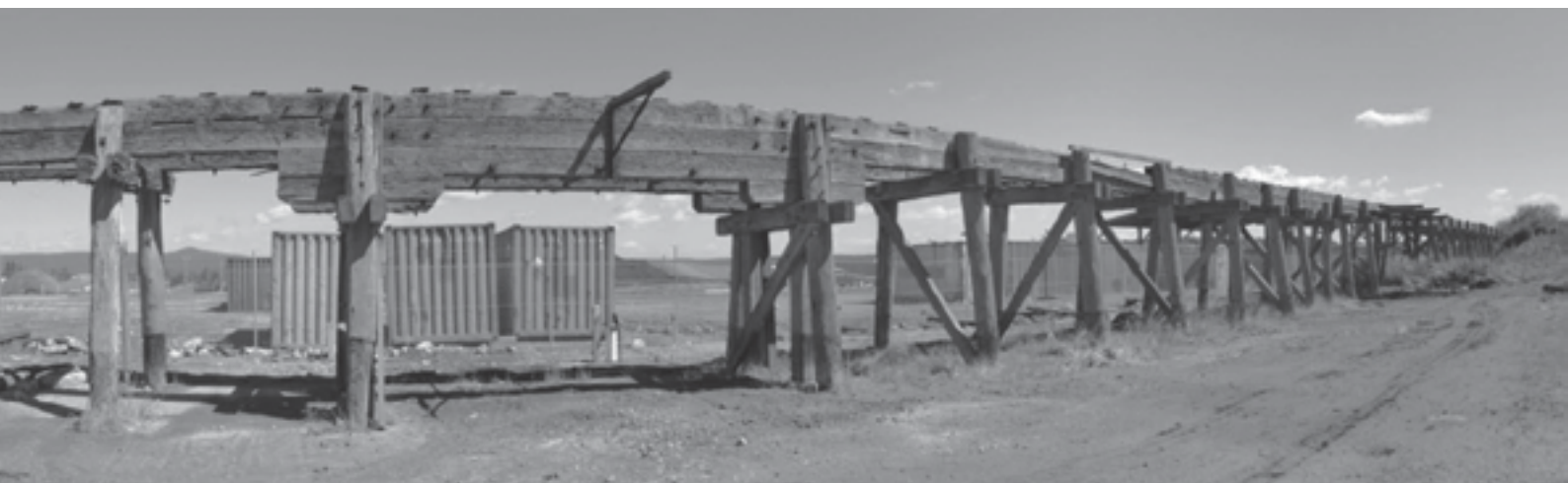
A set of four photographs combined to form a panorama of the railway trestle at Incitec, Boolaroo just prior to its demolition in 2009.
