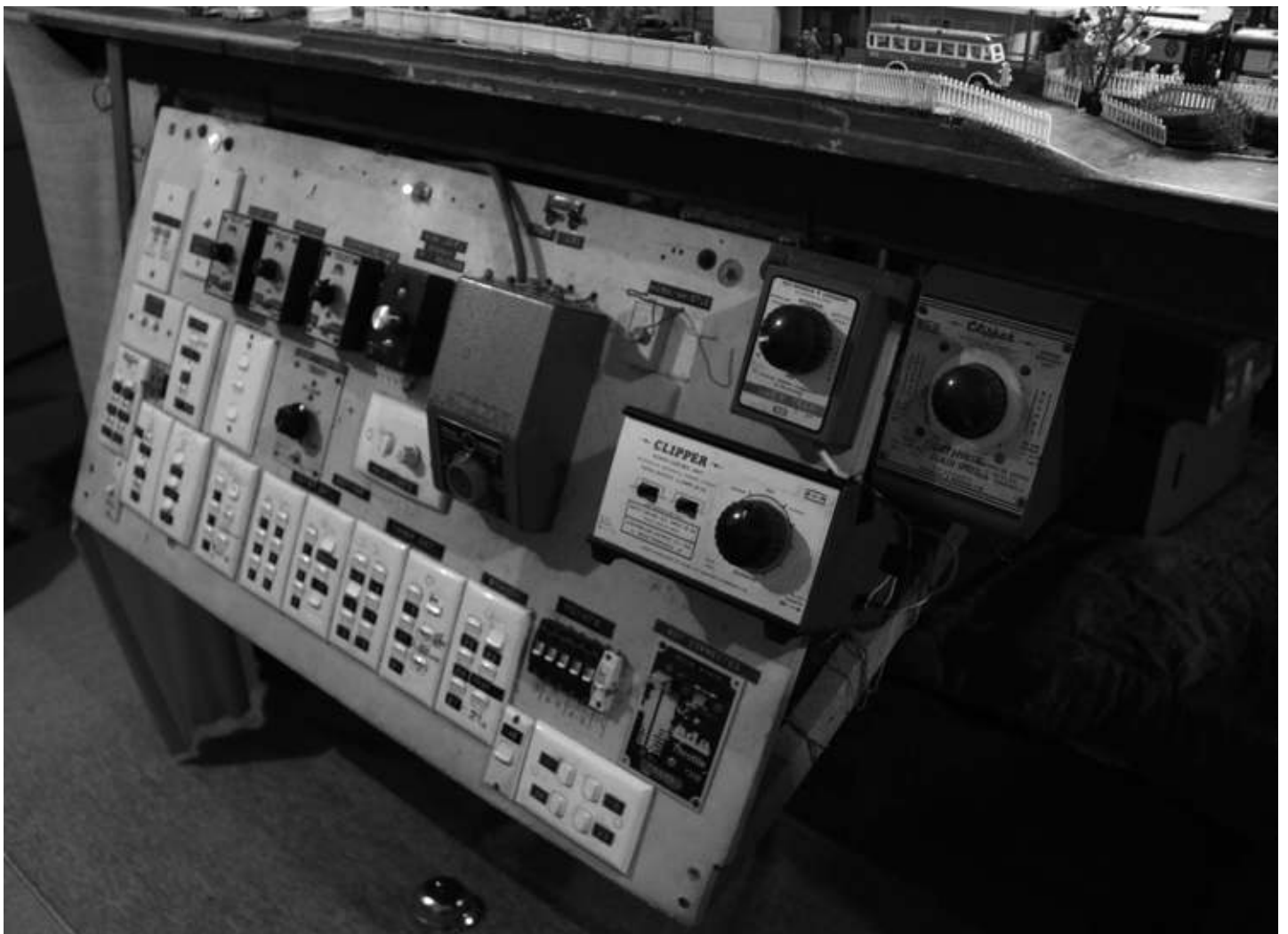
The business end of the layout with the switches, controllers and lighting controls
