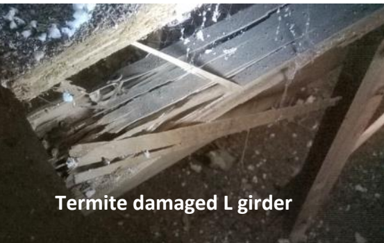
Termite damaged layout leg
