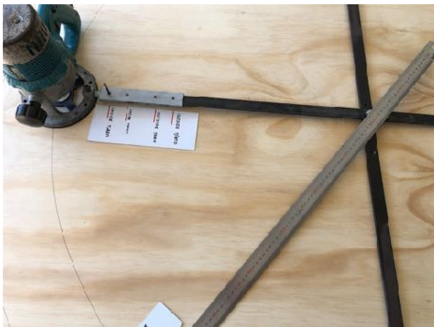
4 Router set up to cut inside trackbed
