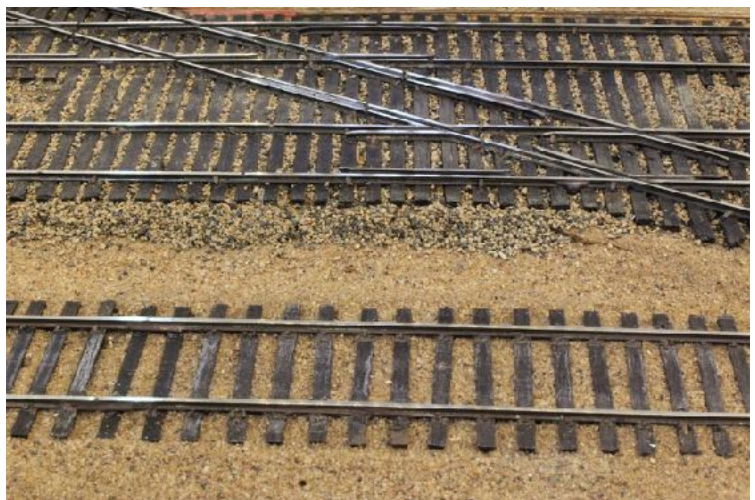
17 The dual diamond crossings in Trevson yard needed to be hand laid as a curved entry was required and there were no commercially available crossings that would fit in this tight space.
