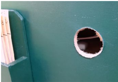
4 A 25mm hole drilled into the Fascia for the plastic Plug
