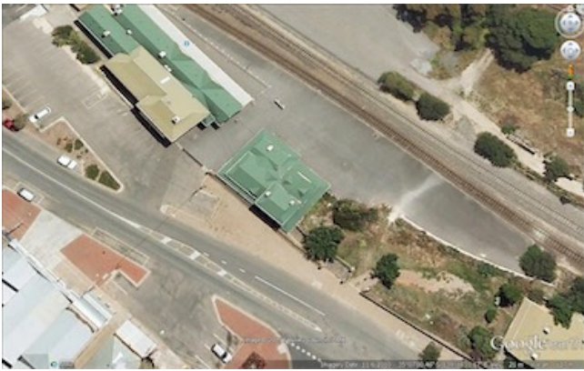
24 Satellite image of station buildings
