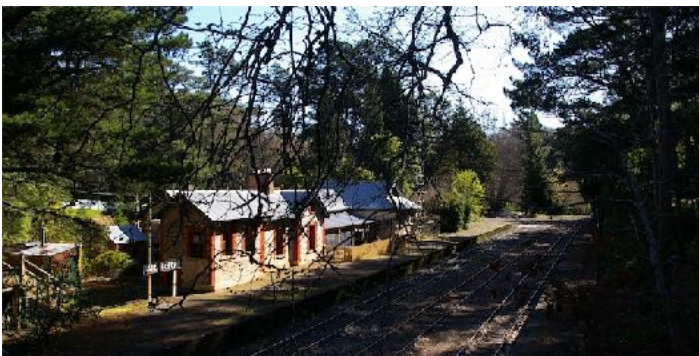
17 Details of the station buildings
