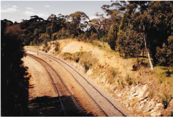
38 Cutting near Belair station
