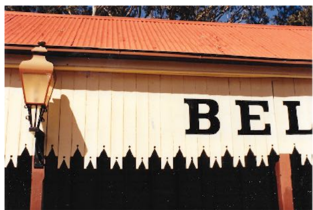
12 Detail of the waiting shed
