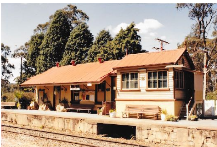
8 Photograph of station building and signal box
