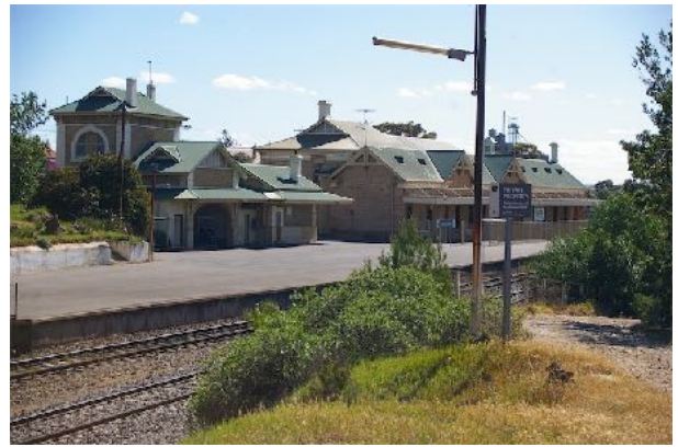
25 General view of station buildings
