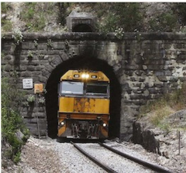
40 Tunnel near Mt Lofty
