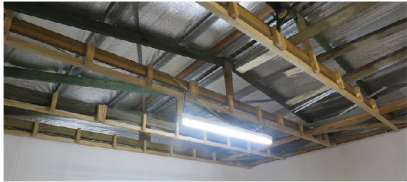
Photo taken showing installation of framework to support ceiling battens
