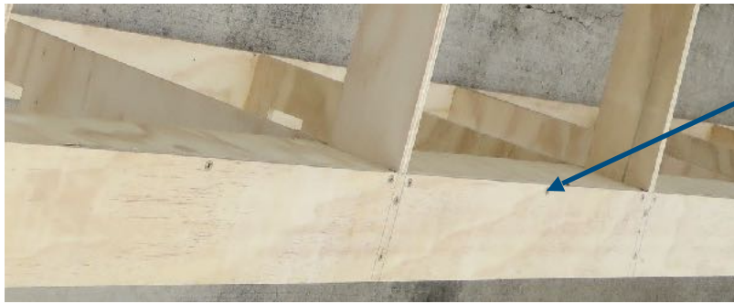
Screws to fasten background support sections
