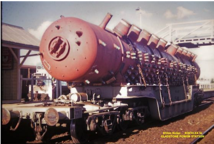
85 ton Gladstone Power House boiler. Photo by Peter Kennedy
