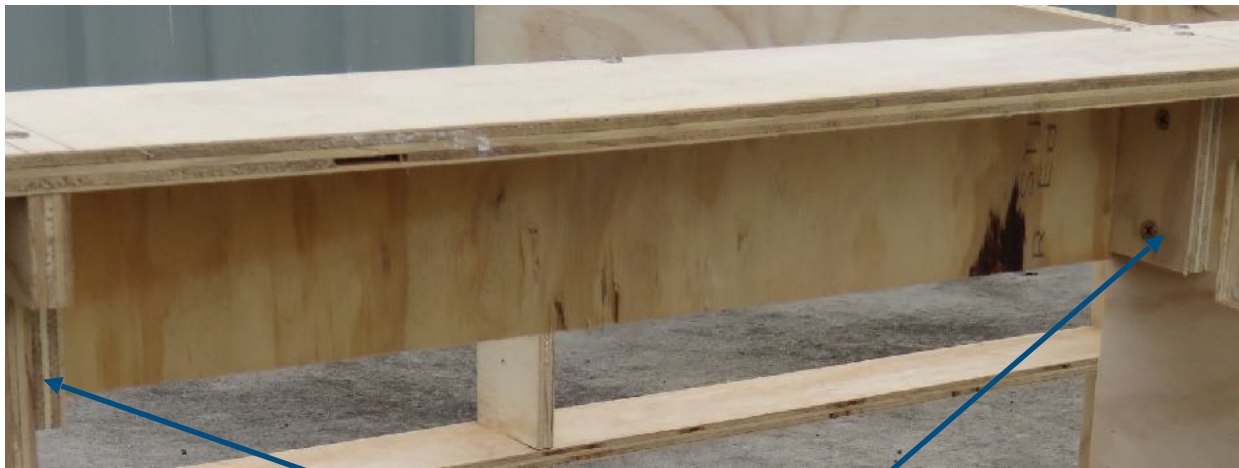
Support blocks screwed into "C section"
