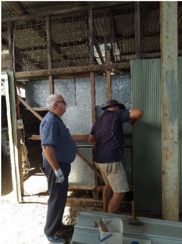
Peter and Steve removing the internal mini orb.
