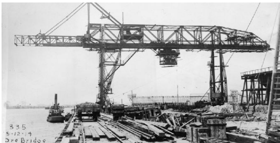
Figure 2 - The Steelworks under construction in 1914, showing an Ore Bridge
