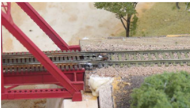
2 Soldered connection of end of guard rail to brass pin drilled into baseboard
