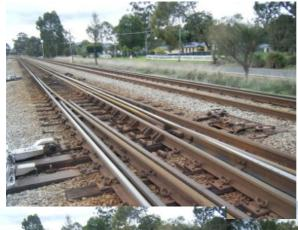
off the double track dual standard gauge (1435 mm) gauge /narrow gauge (1060 mm)
