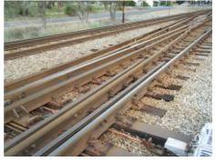
Most of the dual gauge track through the Swan Valley is long length welded rail laid on concrete sleepers.
