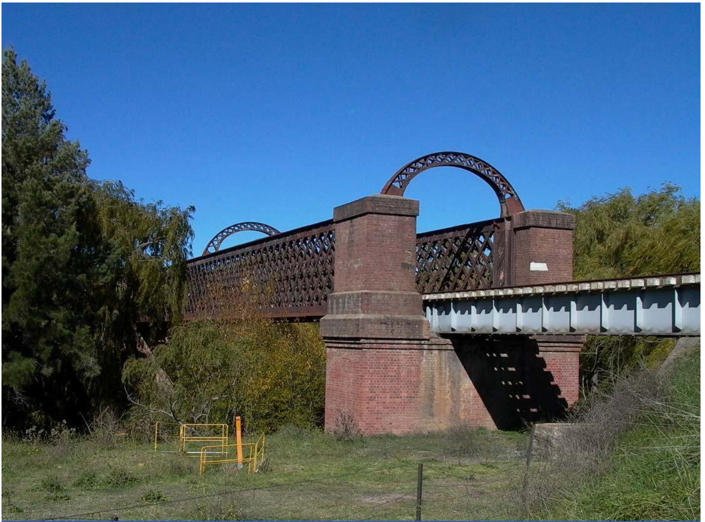
Whitton Lattice Girder Bridge Woolbrook 2012
