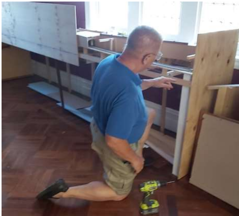
Adding temporary bracing & a back board to strengthen one section from any warping
