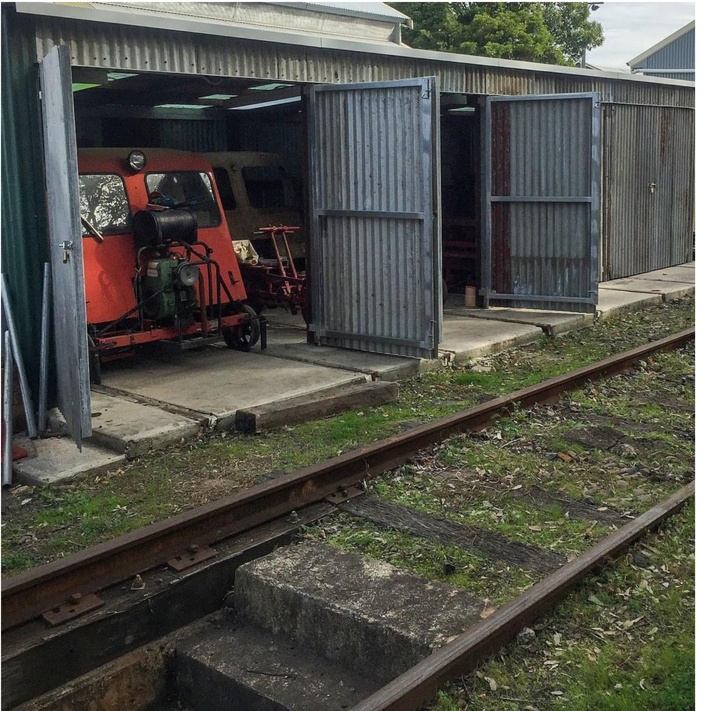
Shed rails set in the concrete, dirt, rocks, weeds amongst the rails & sleepers with a concrete inspection pit!
