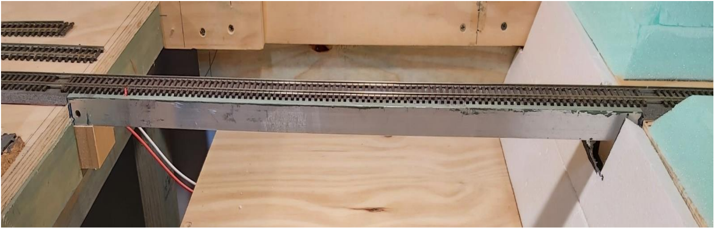
Super elevating the track on the Helix.
