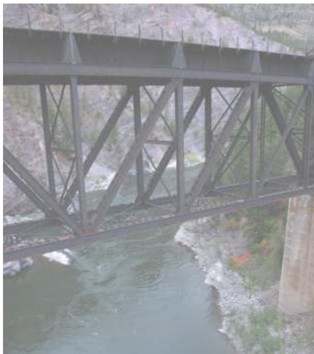
Disused railway bridge
