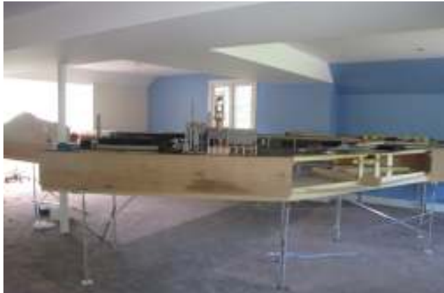
Figure 5: Modules undergoing re-assembly, November 2015
