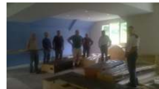
Figure 4: Modules at new location prior to re-assembly
