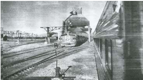
Lamy Cooling Tower over Mainlines
